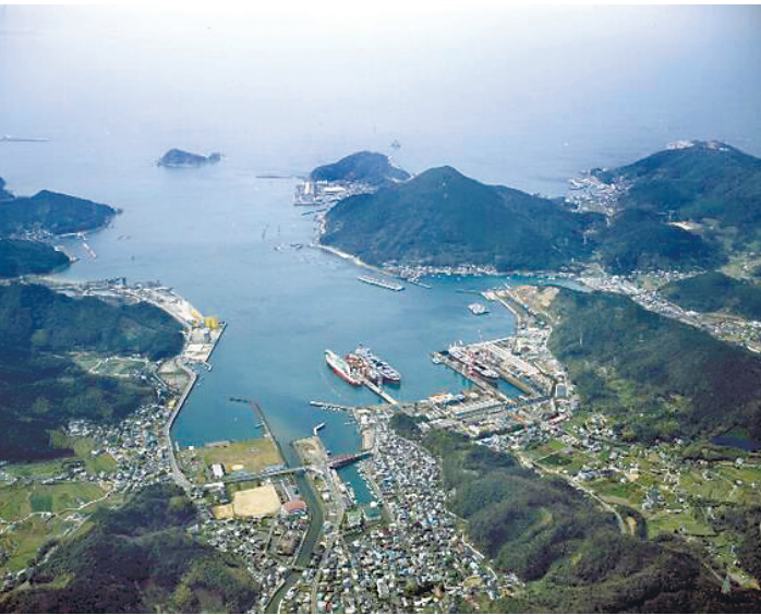
Yura Port in Wakayama Prefecture supports the region’s shipbuilding industry. WAKAYAMA PREFECTURAL GOVERNMENT
