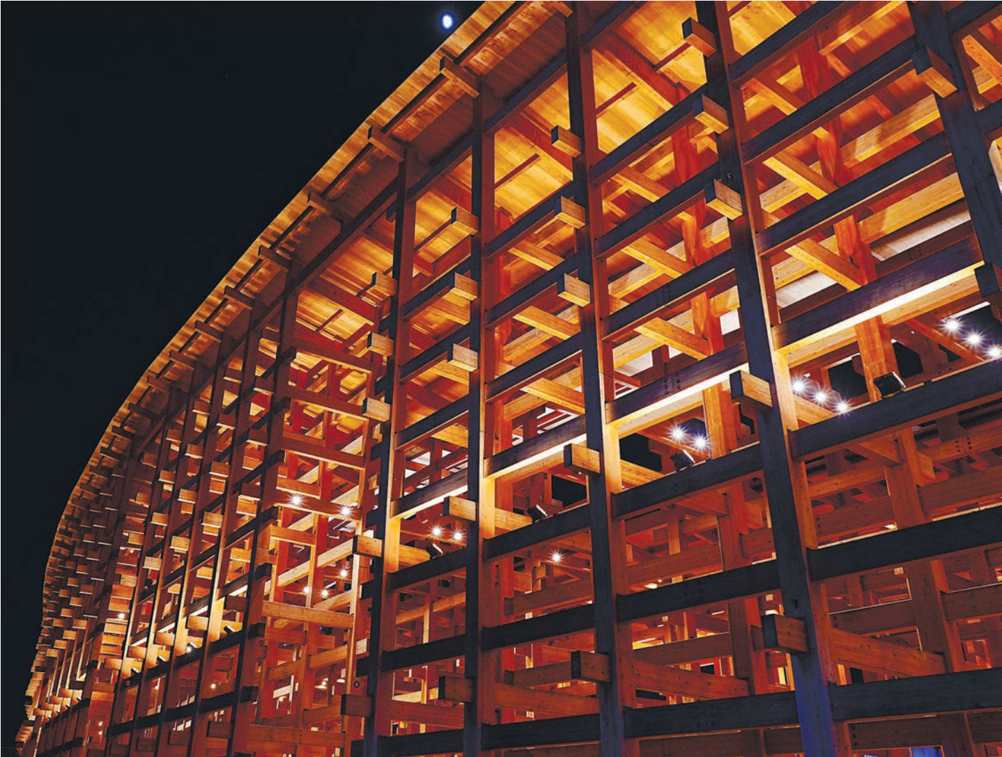
The Osaka Expo's wooden Grand Ring was constructed using traditional construction techniques.
