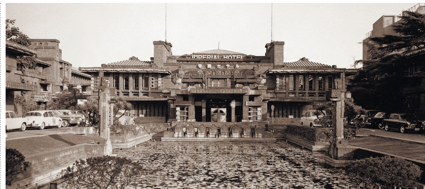
Wright's Imperial, the "Jewel of the Orient," epitomized style, structural mastery and social vibrancy. IMPERIAL HOTEL
