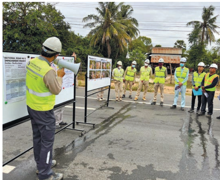
Left: Japanese and Cambodian representatives conduct a final inspection of National Road No. 5 in Kampong Chhnang province in November 2022.
