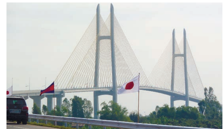
The Japan-funded Tsubasa Bridge spans the Mekong River in Neak Loeng, Cambodia.
