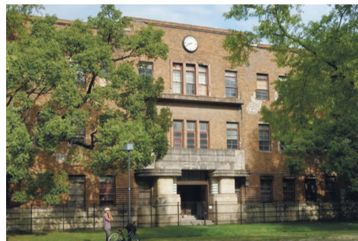
Building No. 1 of the former Faculty of Science, which survived the atomic bombing, is adjacent to the Higashi-Senda Campus. HIROSHIMA UNIVERSITY
