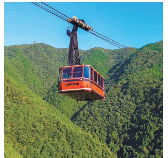
The Unpenji Ropeway offers passengers spectacular scenery as they travel 2.6 kilometers in just seven minutes.
