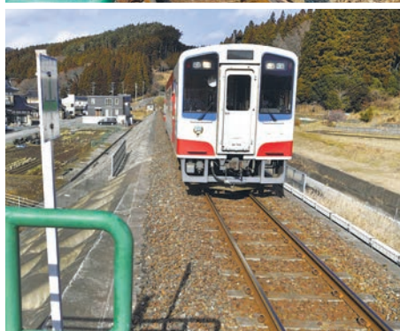
Top: Tsunami debris blocks the Sanriku Railway near Horei Station in Ofunato, Iwate Prefecture, on March 13, 2011. Bottom: A train rolls along the rebuilt tracks in the same area on Jan. 29.
