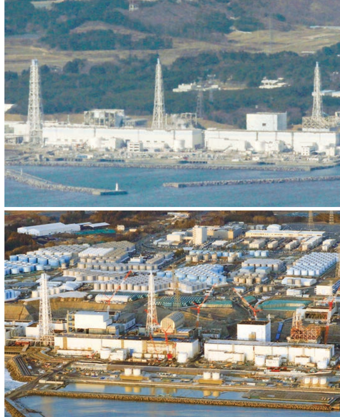
The buildings for reactors 1, 2, 3 and 4 at the Fukushima No. 1 power plant are shown in Fukushima Prefecture on March 17, 2011 (top), and on Feb. 14 with hundreds of tanks in the background holding contaminated cooling water awaiting disposal. KYODO
